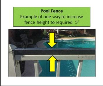
The exterior side of the fence is free of footholds and handholds. The Life Safety Inspector will look around the area and measure 3' from the fence to identify any potential items that could be used as a handhold / foothold or affect the height of the fence such as a change in landscaping.
