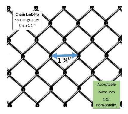
All openings must measure less than 4" (bottom, between slats and all connections)
